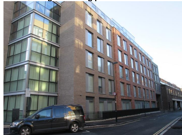
Existing buildings on opposite side of Pear Tree Street
