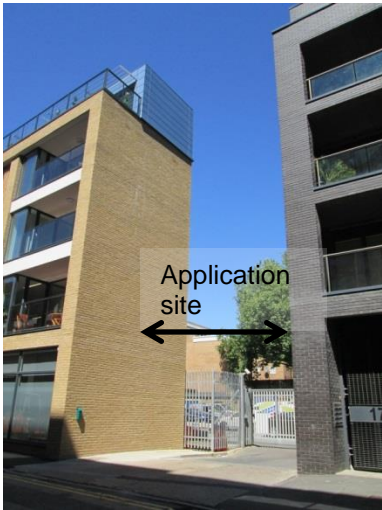
Existing entrance from Pear Tree Street
