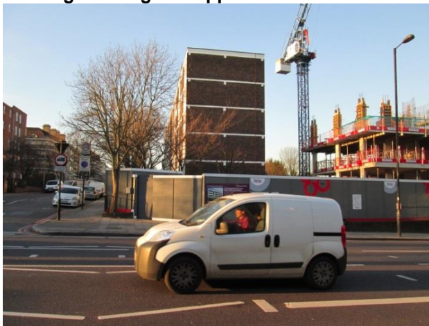
John Barnes Library site (under construction)
